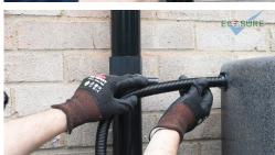
**c.** Tighten the nut on the outside by hand to form a seal.
