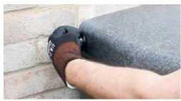
**h.** Push the flexible hose onto both connectors. A small amount of lubricant can help.
