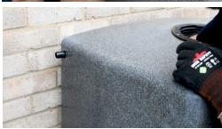
**g.** Measure and cut the diverter hose to length, keeping the pipe straight.
