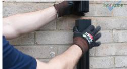
**b.** Push the connector through the hole with the washer on the **INSIDE**
